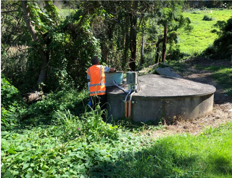
Photo 5: Leachate collection chamber to the south of landfill footprint / adjacent to Raupo Swamp.
